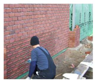
For inside corners, cut bricks minimum 3 5/8" long are positioned adjacent to a full brick as per drawing. This is then alternated on each course to achieve the effect of a traditional brickwork construction.
